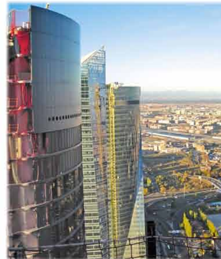
Diverse scaffold for the construction of the Resol Tower, Madrid, Spain
