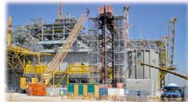
Diverse scaffold for the construction of the LNG Adriatic, Algeciras, Spain
